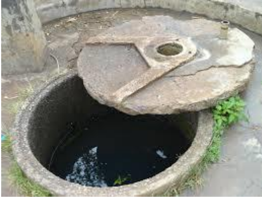
The latest picture of the water and sanitation project
