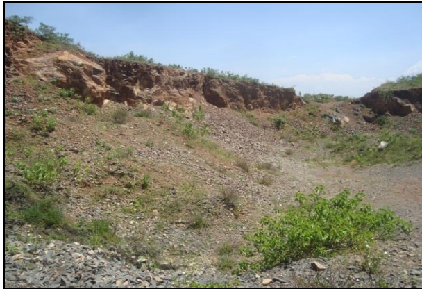
Plate 4.12: Part of the Kanyawegi site showing the exposed rugged walls. Source: Author. (October, 2016).
