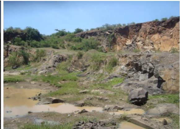
Plate 4.13: Rugged high stone walls at Wathorego post-mine site and waterlogging within the deepest end of the pit. Source: Author
