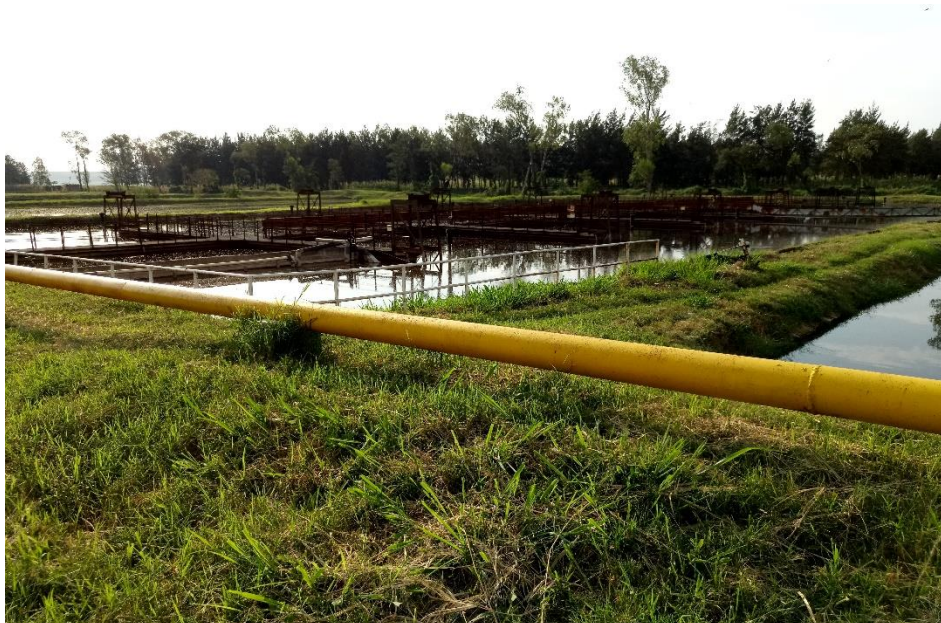
Figure 21; A Sewer treatment plant, owned by Agro-Chemicals
