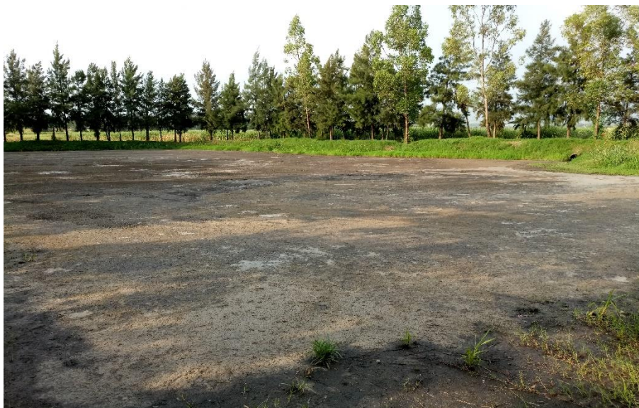
Figure 20; Sewer treatment Pond by MUSCO. Popularly known as Lagoon
