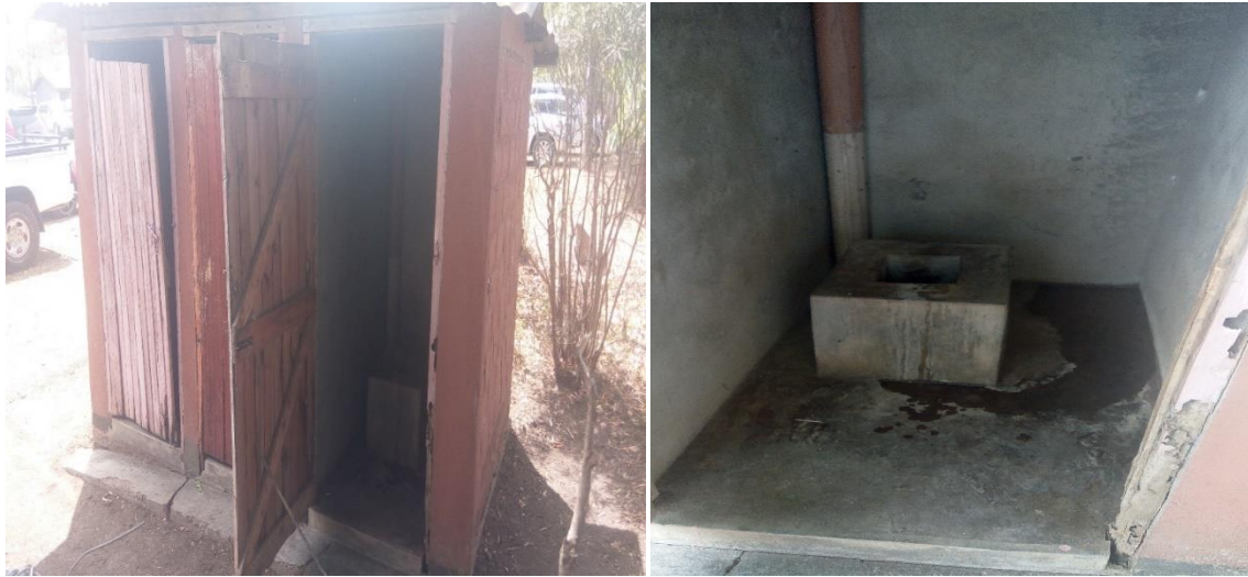
Figure 17: Improved pit latrine with Vent and squatting pan at Sondu town
