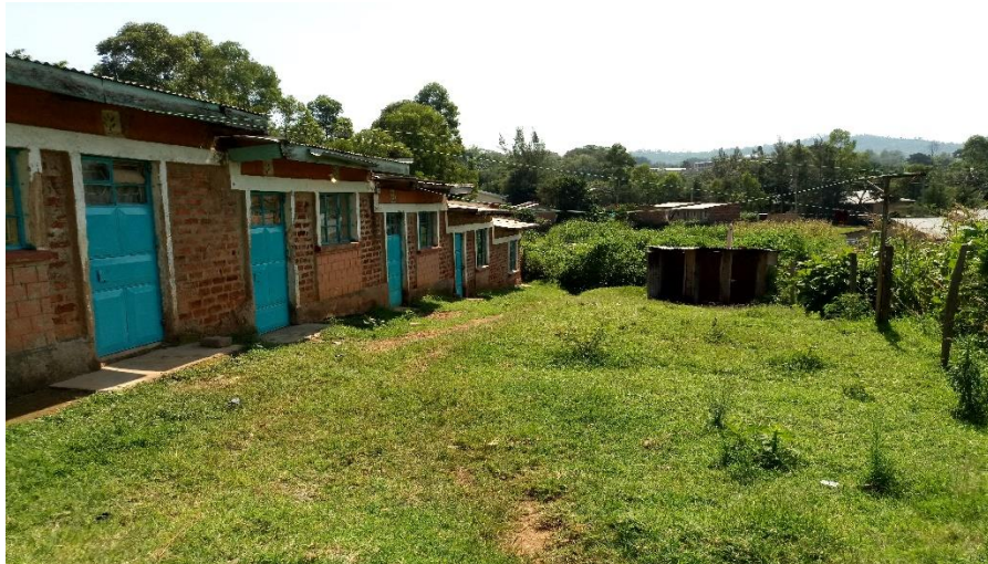
Figure 9: Shared pit latrine in Maseno Town
