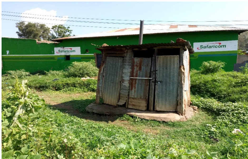
Figure 16: A pit latrine in Maseno constructed using iron sheets
