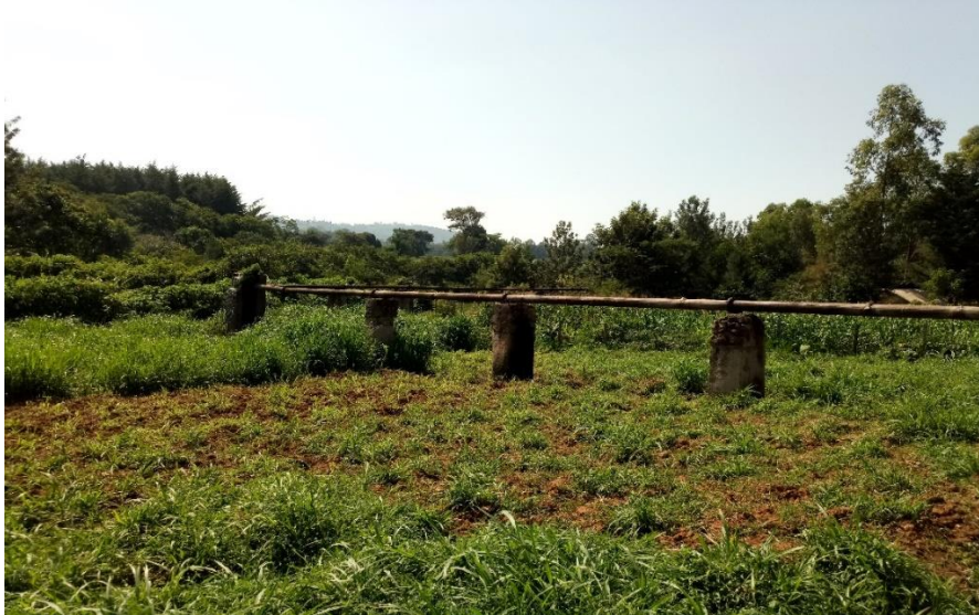
Figure 19: Reticulated Sewer Line in Maseno town
