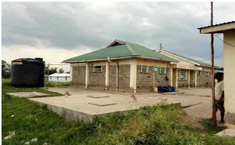
Figure 23: Public Sanitation in Muhoroni town (flushing to a septic tank)
