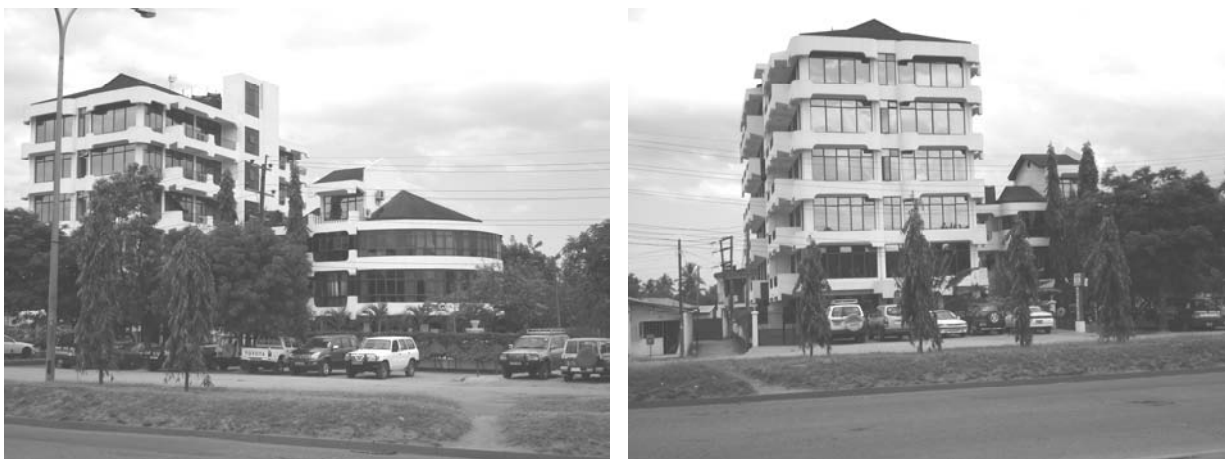
Figure 6-25: Views of the Landmark Hotel from Mandela Rd.
