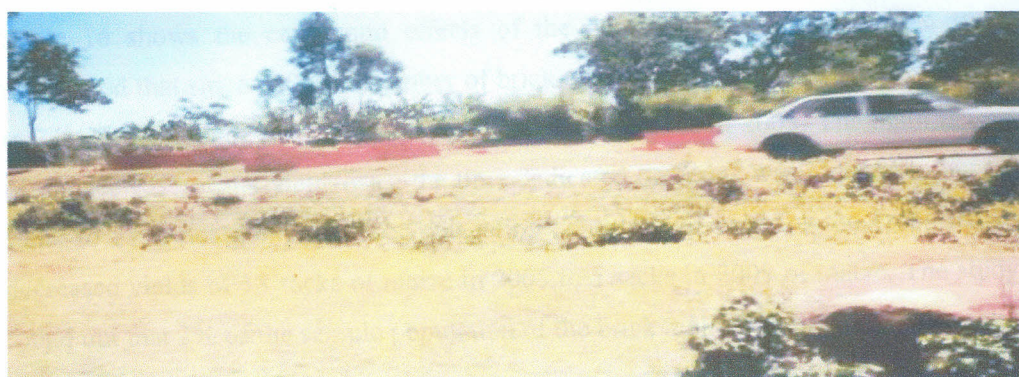
Plate 11: Bricks along road reserve ready for transportation.
