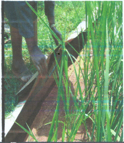
gutter channels directing runoff water into the PVC tanks
