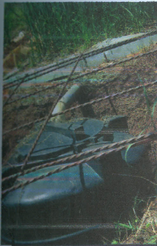
PVC tank placed in close out hole
